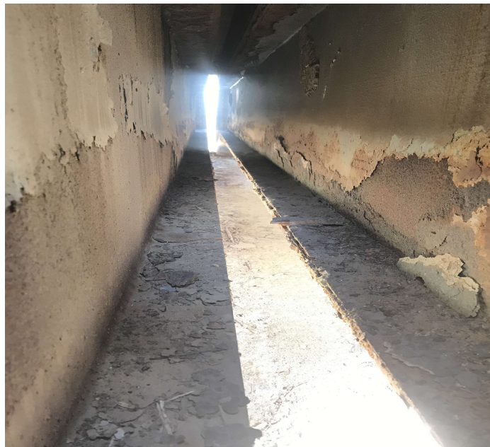
PHOTO 4 Description Floor beams over Bent # 3. Left side. Active corrosion.
