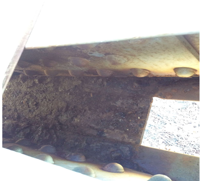
PHOTO 2 Description Span # 2 L3-L4 Right section loss in the lower chord splice.
