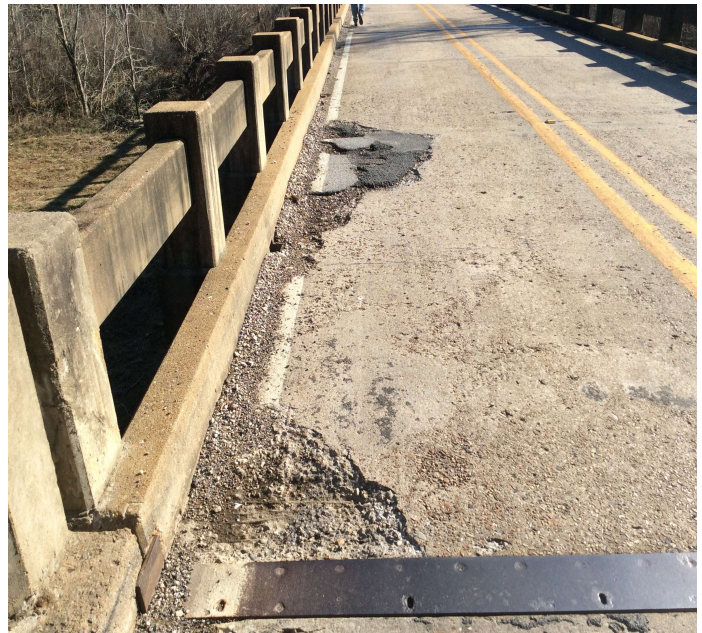
PHOTO 2 Description Span # 5 spalling with exposed reinforcing steel.
