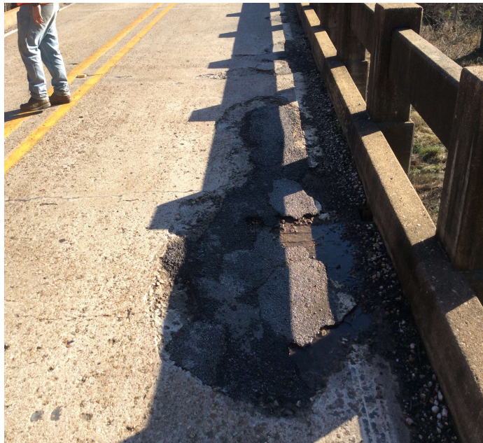
PHOTO 1 Description Span # 5 spalling with exposed reinforcing steel.
