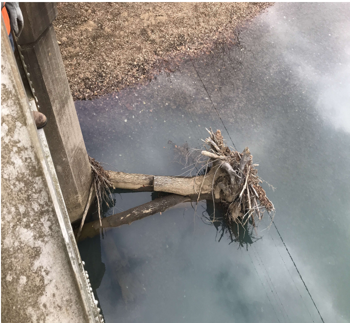
PHOTO 1 Description Inlet Bent # 2. Drift.
