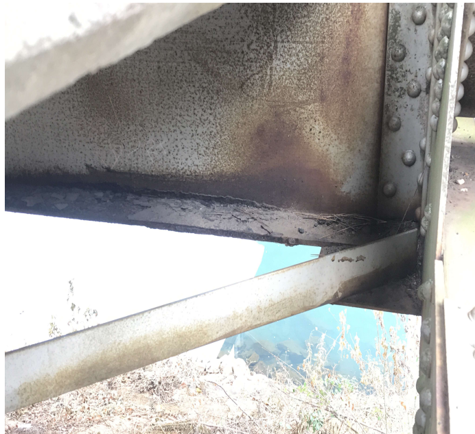
PHOTO 1 Description Span # 1 Right. L2 floor beam corrosion.
