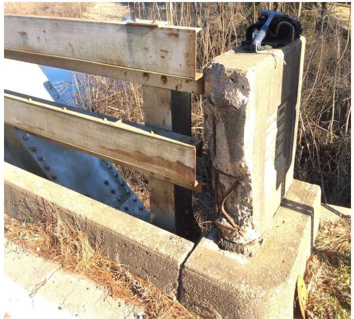
PHOTO 2 Description End post at Bent 1 Rt has collision damage with exposed rebar.
