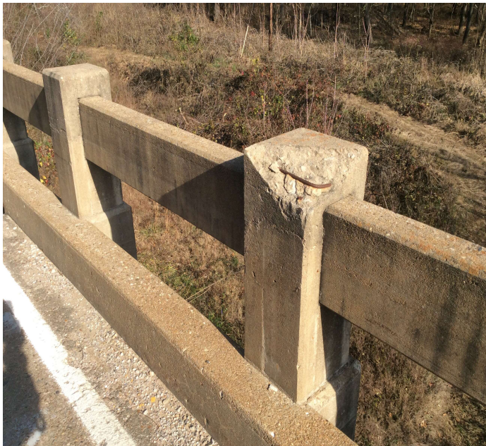
PHOTO 1 Description Span # 4 Rt. Post # 7 has collision damage.
