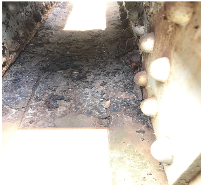
PHOTO 6 Description Span # 3. Right. L3-L4. Lower chord.
