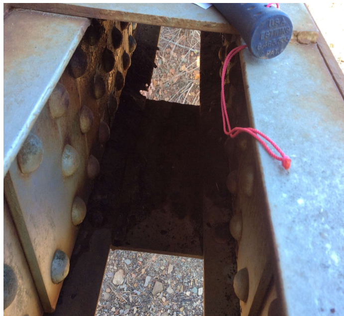
PHOTO 1 Description Span # 2 L1-L2 Right with a 3/4" & a 1/4" hole rusted through the interior lower chord.
