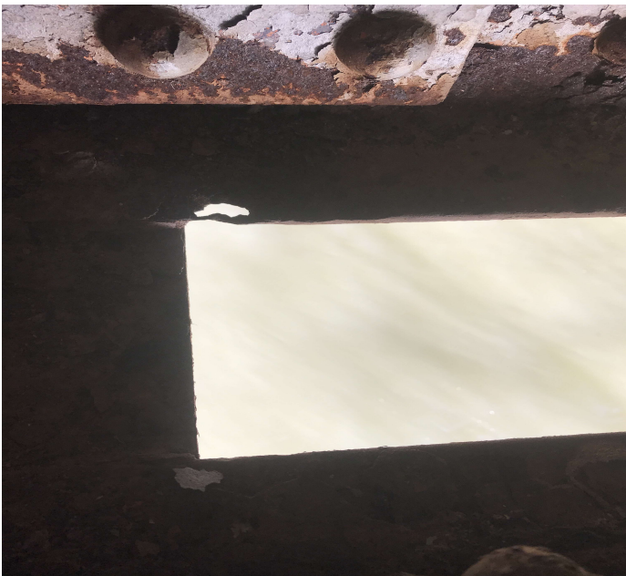
PHOTO 8 Description 1" hole L9-L10 splice.
