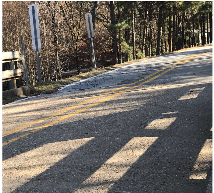
PHOTO 2 Description Asphalt settlement at the South bridge end.
