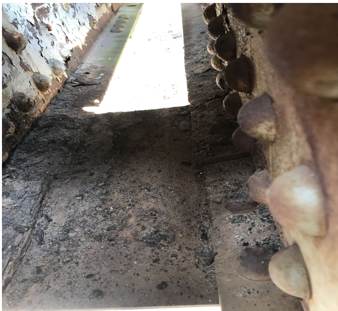
PHOTO 4 Description Span # 2 right. L1-L2. Lower chord. Corrosion.
