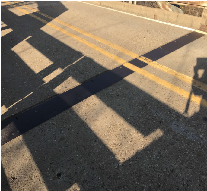
PHOTO 1 Description Sliding plate over Bent # 3.
