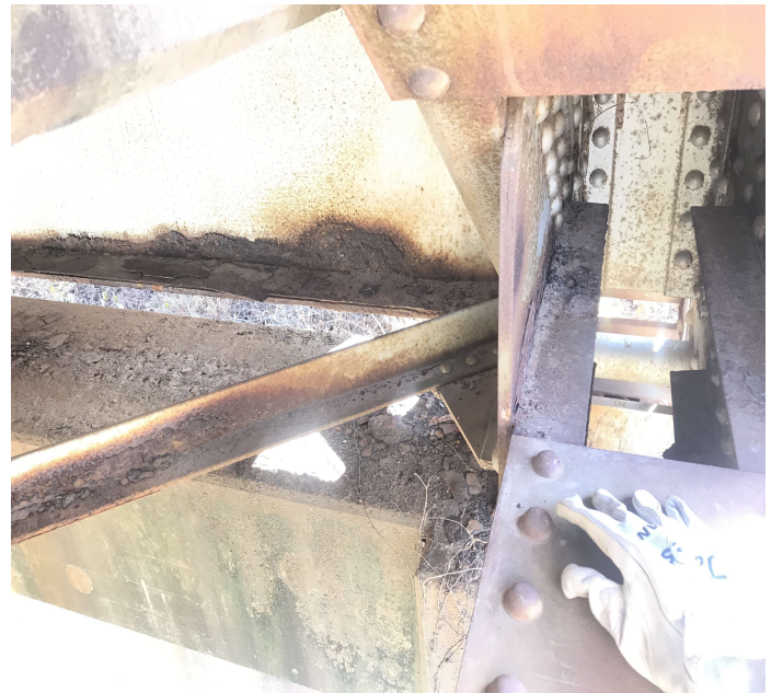
PHOTO 5 Description Span # 3 Left. L0 Corrosion in connection and in the bottom flange of the floor beam.
