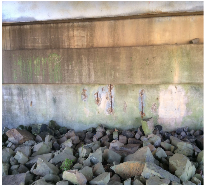
PHOTO 2 Description Bent 1 has 4 vertical spalls with exposed reinforcing steel. Exposed reinforcing steel has initial section loss at this inspection.
