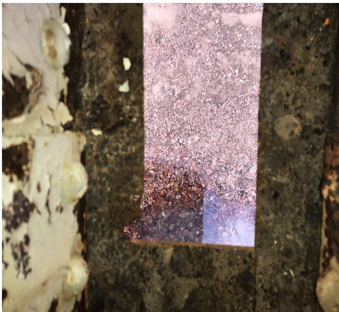
PHOTO 3 Description Span # 2. Right side. 3/4" hole; Section loss. Interior Channel. Splice; L1-L2 Bottom chord.
