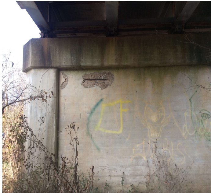
PHOTO 1 Description Bent 5 Span 4 has a 3' spall with exposed reinforcing steel and initial section loss in the web wall
